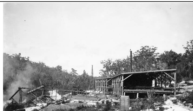
McKenzie's sawmill operations 1918-1922. Logs were delivered to the top of the mill (right of photo) by locomotives, processed into sawn timber that emerged at the bottom of the mill (left) to be conveyed to McKenzies Jetty by locomotives
